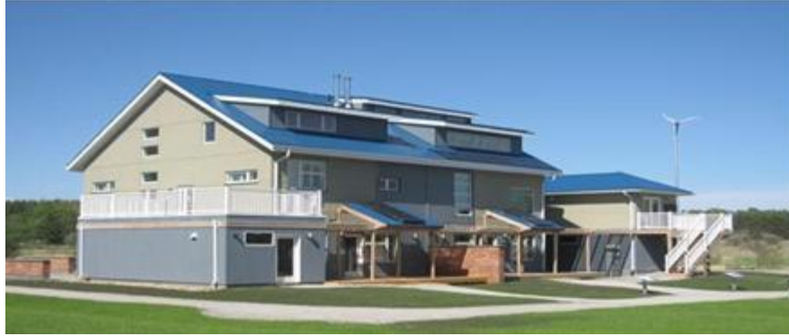
Figure 1. South-west side of twin houses
